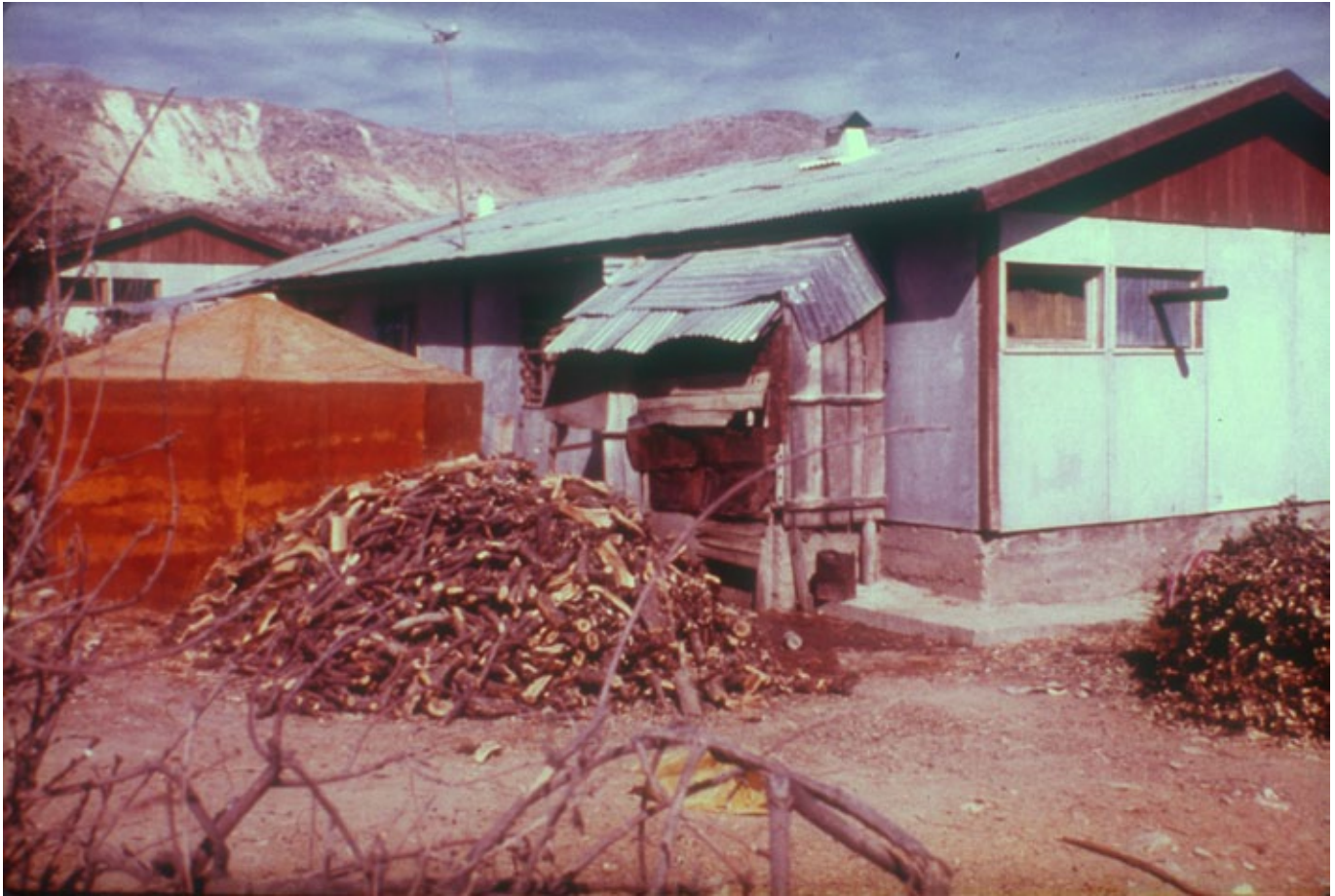
This picture illustrates three types of disaster assistance following the Lice earthquake in Turkey, 1975. On the right, a pre-fabricated house as provided by the Turkish government; on the left an emergency shelter made of polyurethane provided by OXFAM; and in the centre, an improvised addition to the house made by occupants. Many families objected to the form and siting of the housing. These objections related to their lack of participation in what was provided, and the cultural and climatic unsuitability of the housing. OXFAM used their polyurethane house for the first and only time. Four hundred and sixty-three units were produced.
